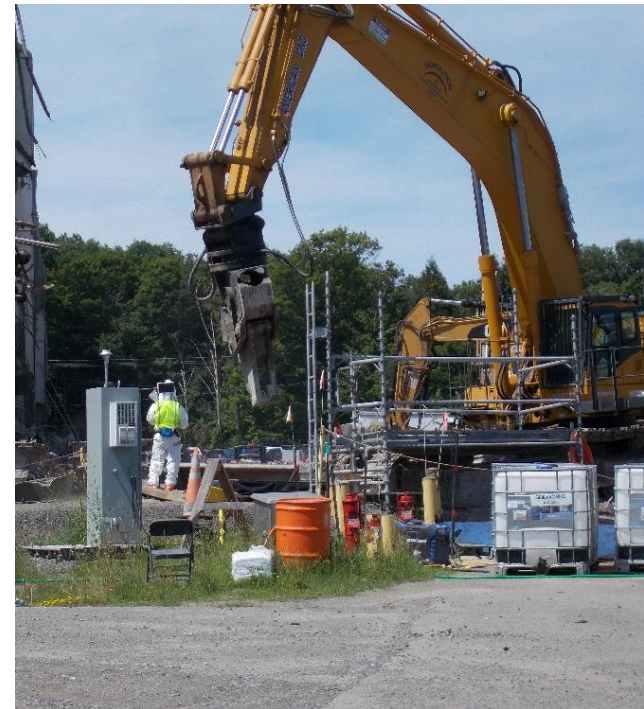
RCT performs monitoring during demolition activities
