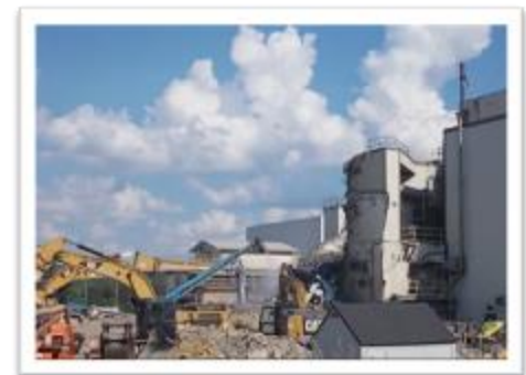
Vitrification Facility demolition
